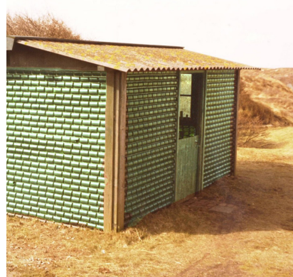
Pictures of the prototype of the WOBO bottle and a house made of the bottles. Available at: https://www.heinekencollection.com/stories/the-story-behind-the-wobo/
